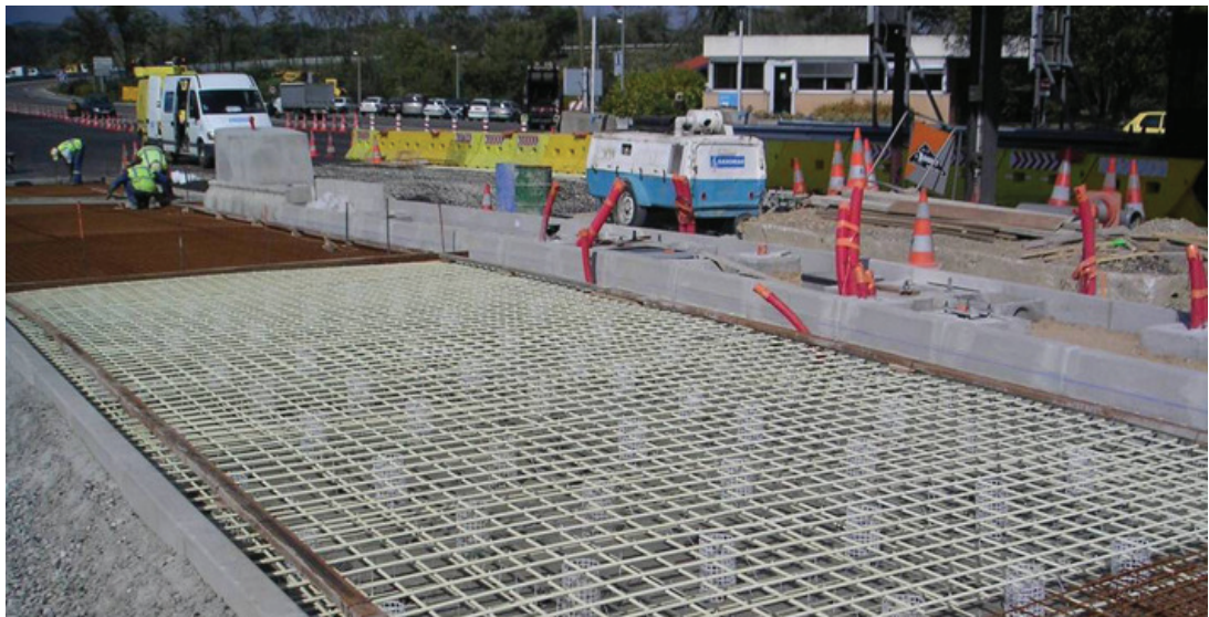
Replacement of the carriageway slab ,Péage de Tain, France
