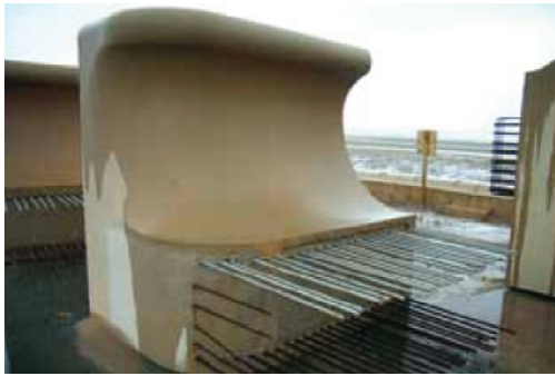
Precast concrete elements for coastal defense project blackpool, UK
