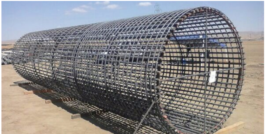
Reinforced concrete pipe for waste water transmission, Tehran, Iran
